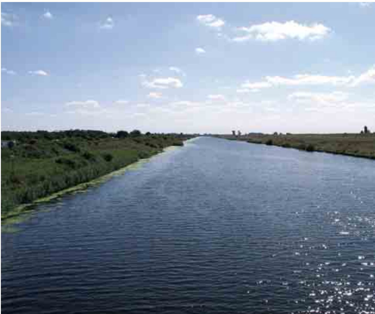
Flood Relief Channel
