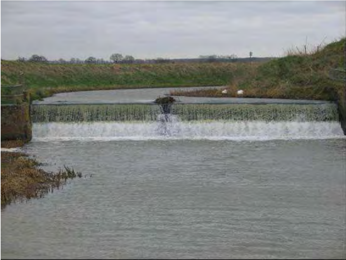
Plate 57 Harlam Hill Weir (d/s) on the River Ancholme (source: HIFI)
