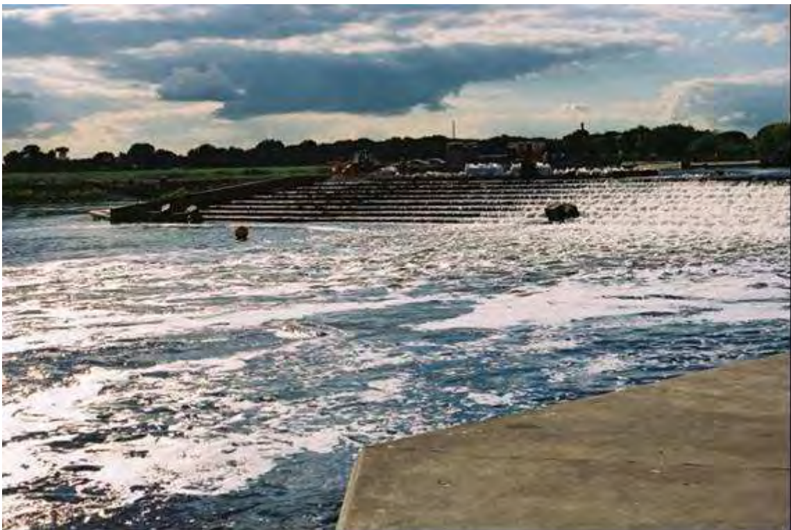
Plate 34 Beeston Weir on the River Trent (source: Trent Rivers Trust)
