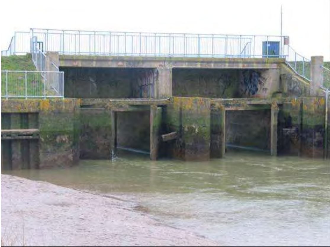
Plate 65 The tidal barrage on Tetney Haven near Stonebridge Farm (source: HIFI)
