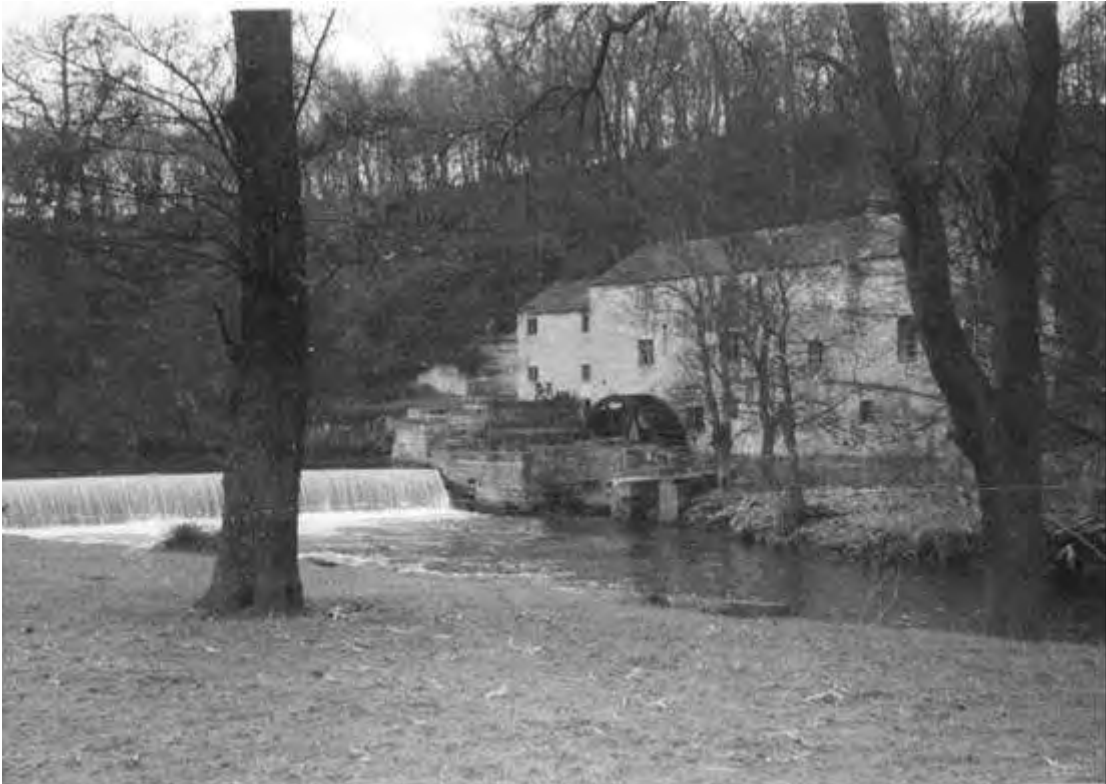
Plate 24 Flint Mill Weir on the River Wharfe (source: Environment Agency)
