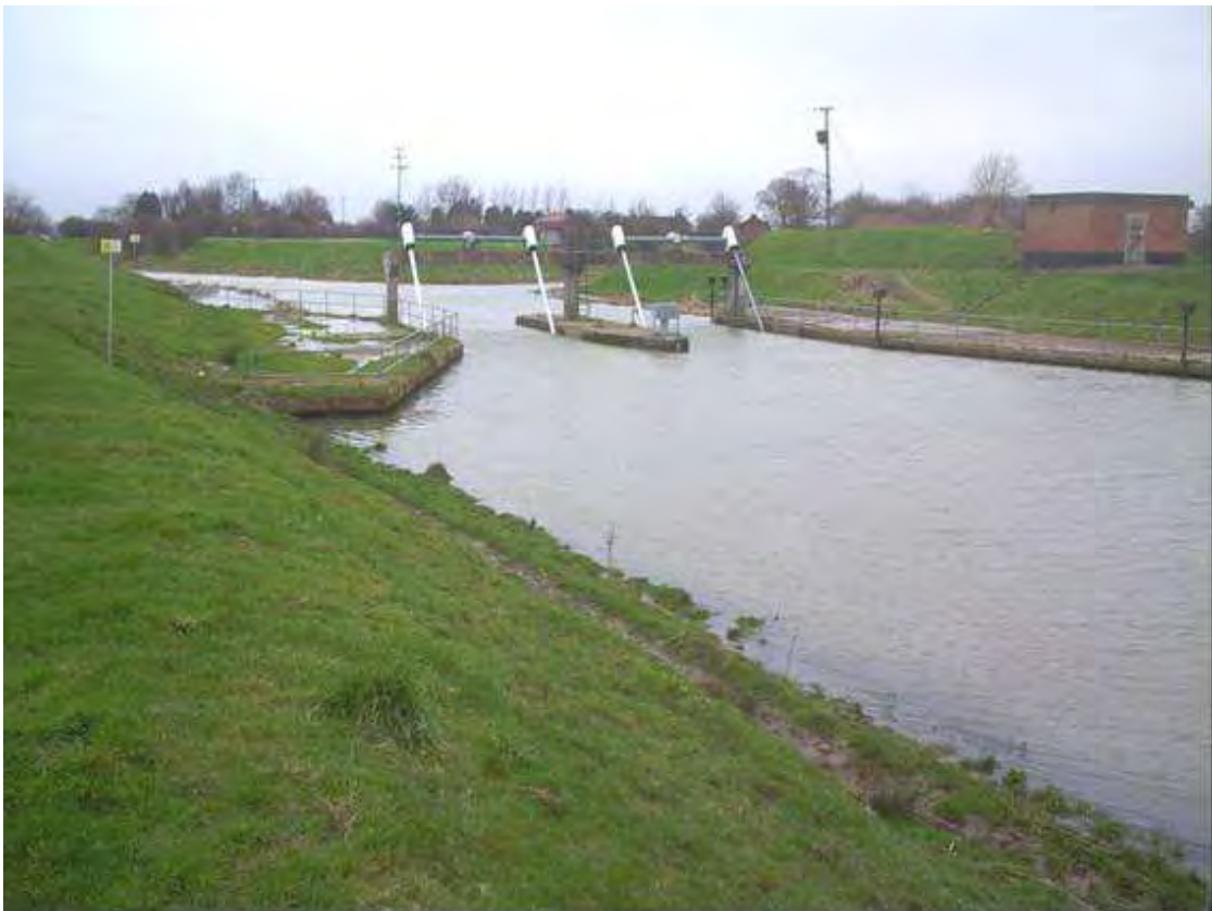
Plate 66 The weir at Tetney Lock on Tetney Haven (source: HIFI)
