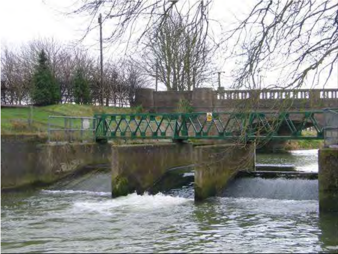
Plate 59 Bishopbridge Weir on the River Ancholme (source: HIFI)
