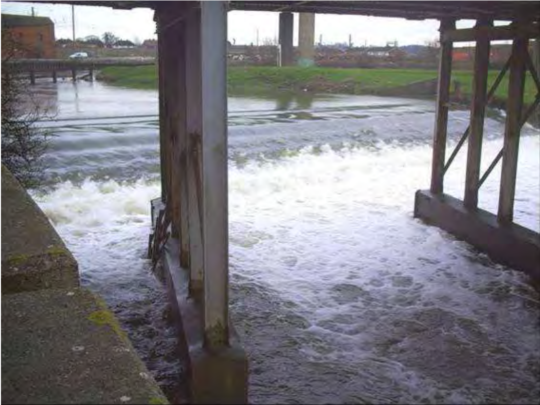
Plate 27 Nether Lock Weir on the River Trent (source: HIFI)
