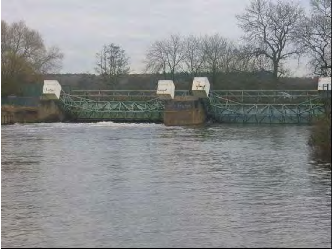
Plate 7 Elvington Weir on the Yorkshire Derwent (source: HIFI)
