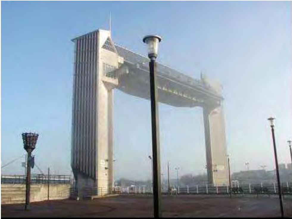
Plate 1 The tidal barrage at the mouth of the River Hull (source: Environment Agency)
