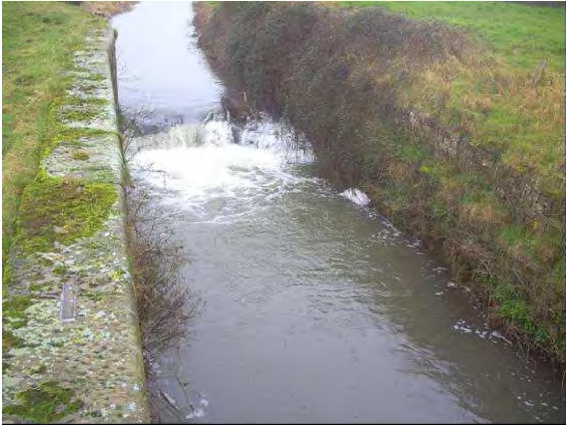
Plate 67 Alvingham Weir on Tetney Haven (source: HIFI)
