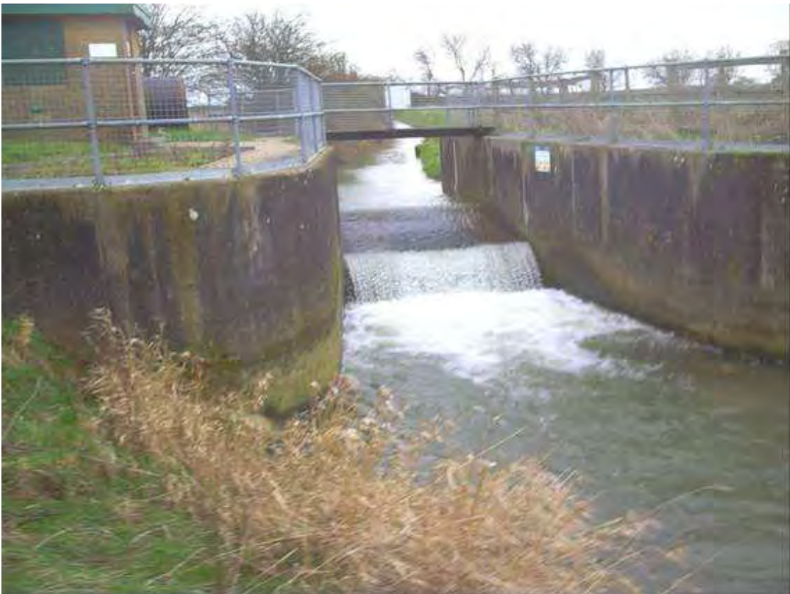
Plate 60 Toft Newton Weir on the River Ancholme (source: HIFI)
