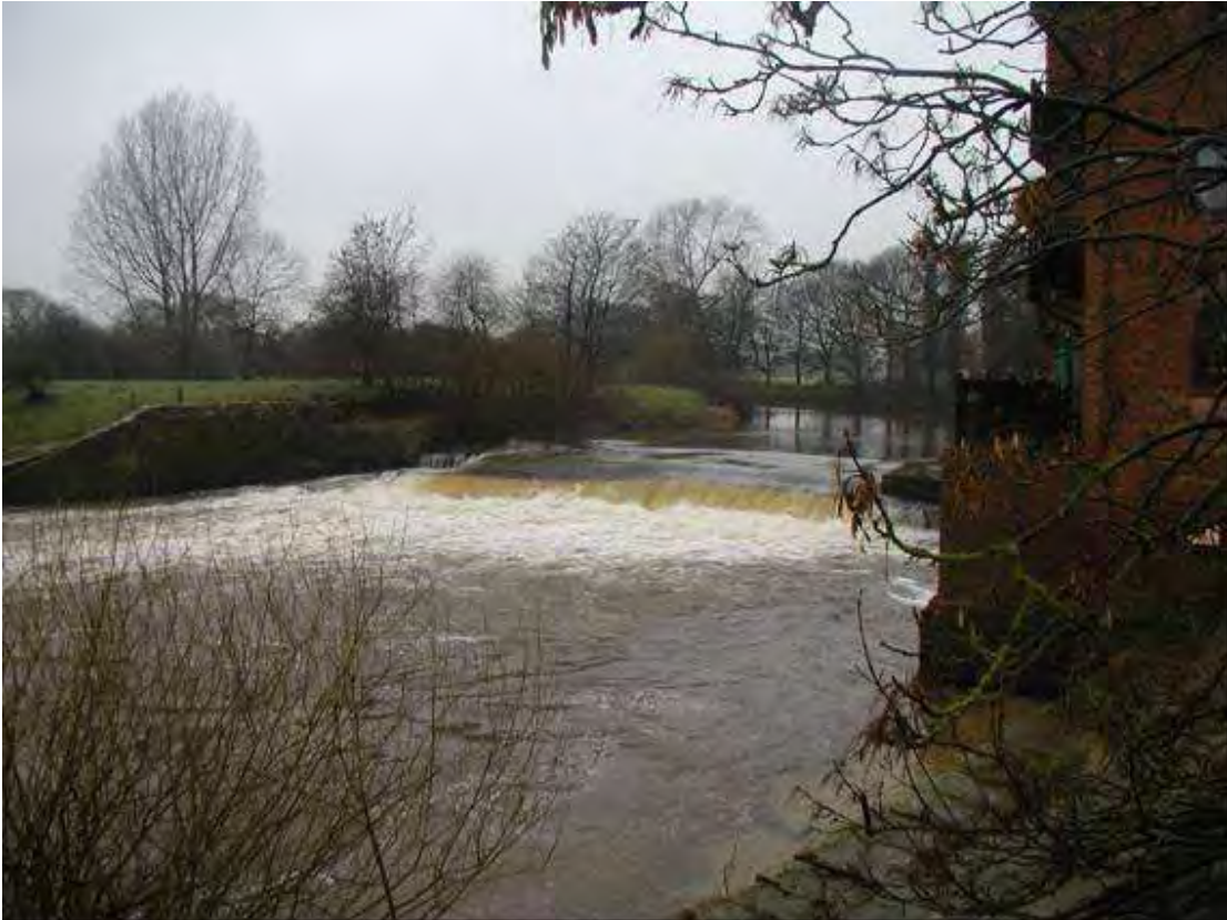
Plate 16 Topcliffe Weir on the River Swale (source: Environment Agency)
