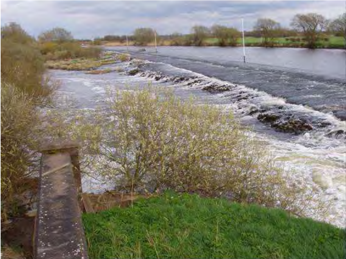
Plate 28 Averham Weir on the River Trent (source: Environment Agency)
