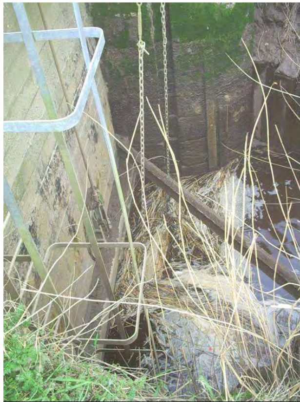
Plate 64 The outfall of Swinefleet Warping Drain at Swinefleet (source: HIFI)
