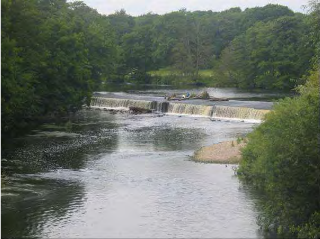
Plate 23 Boston Spa Weir on the River Wharfe (source: HIFI)
