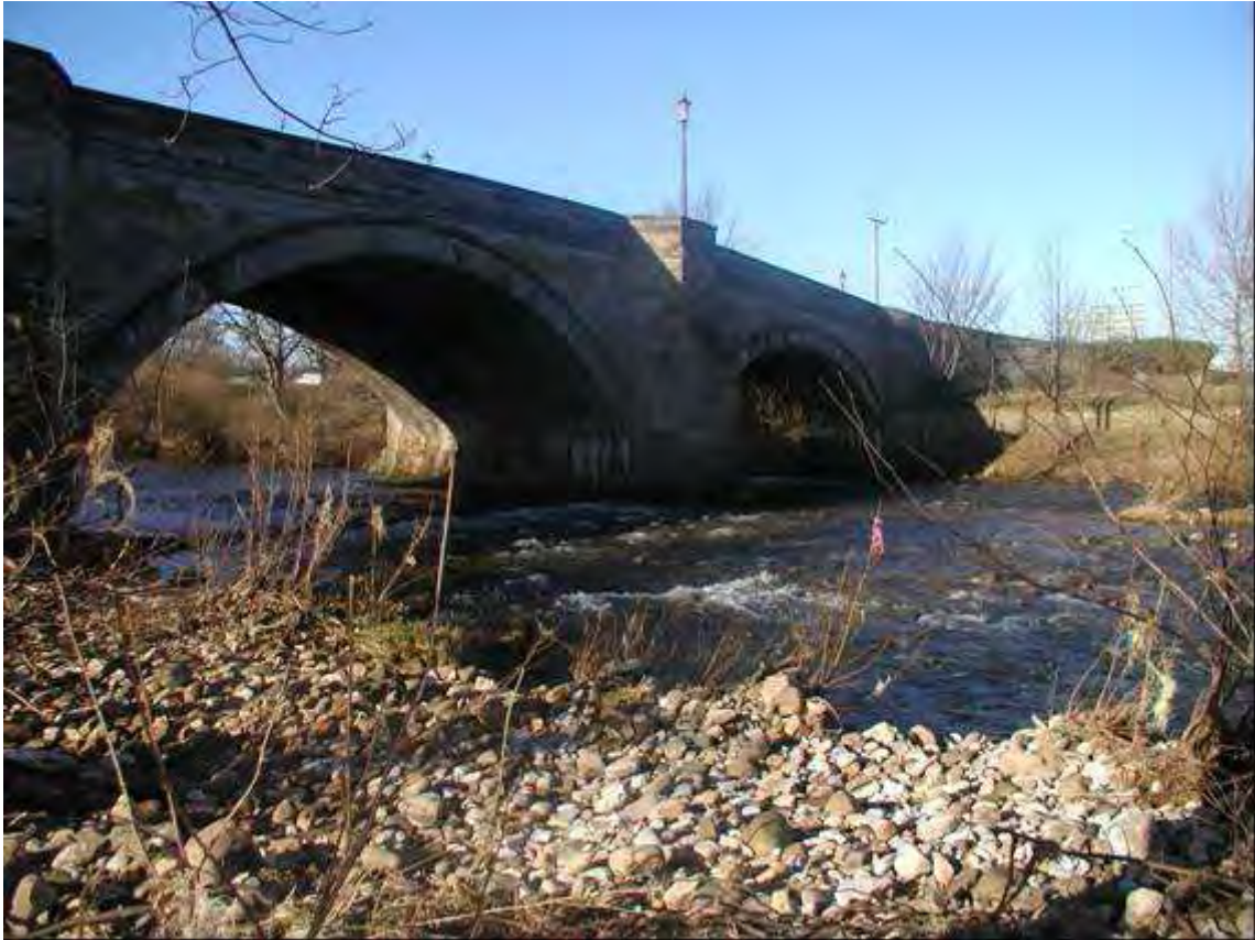
Plate 17 Catterick Bridge on the River Swale (source: Environment Agency)
