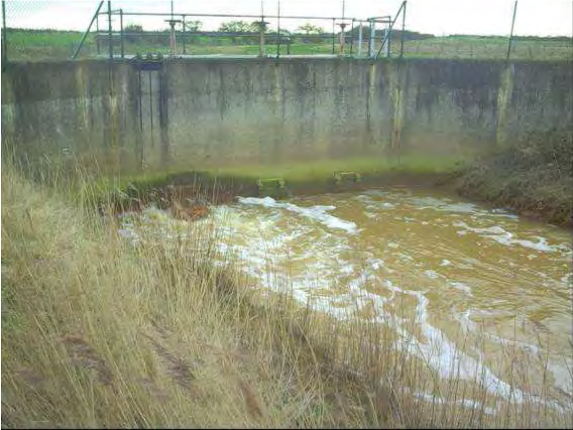
Plate 69 The sluice at Cow Lane on Adlingfleet Drain (source: HIFI)
