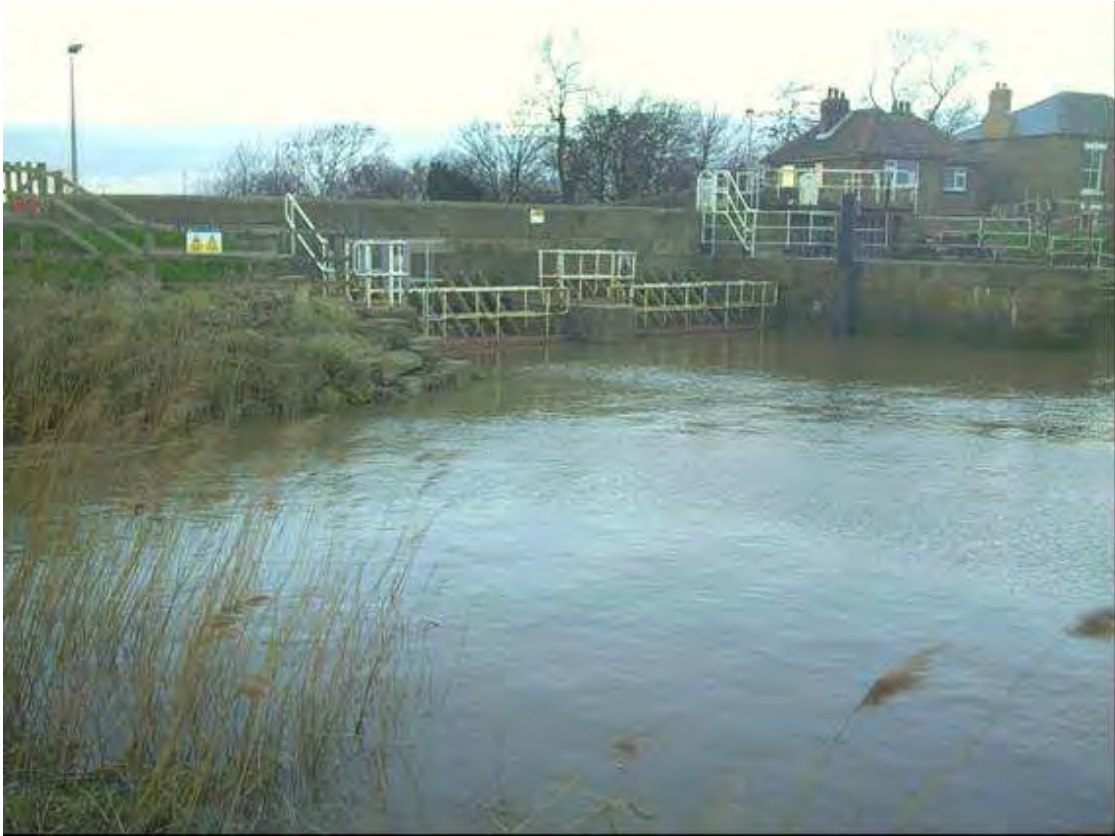
Plate 61 Weighton Lock on the River Foulness/Market Weighton Canal (source: HIFI)
