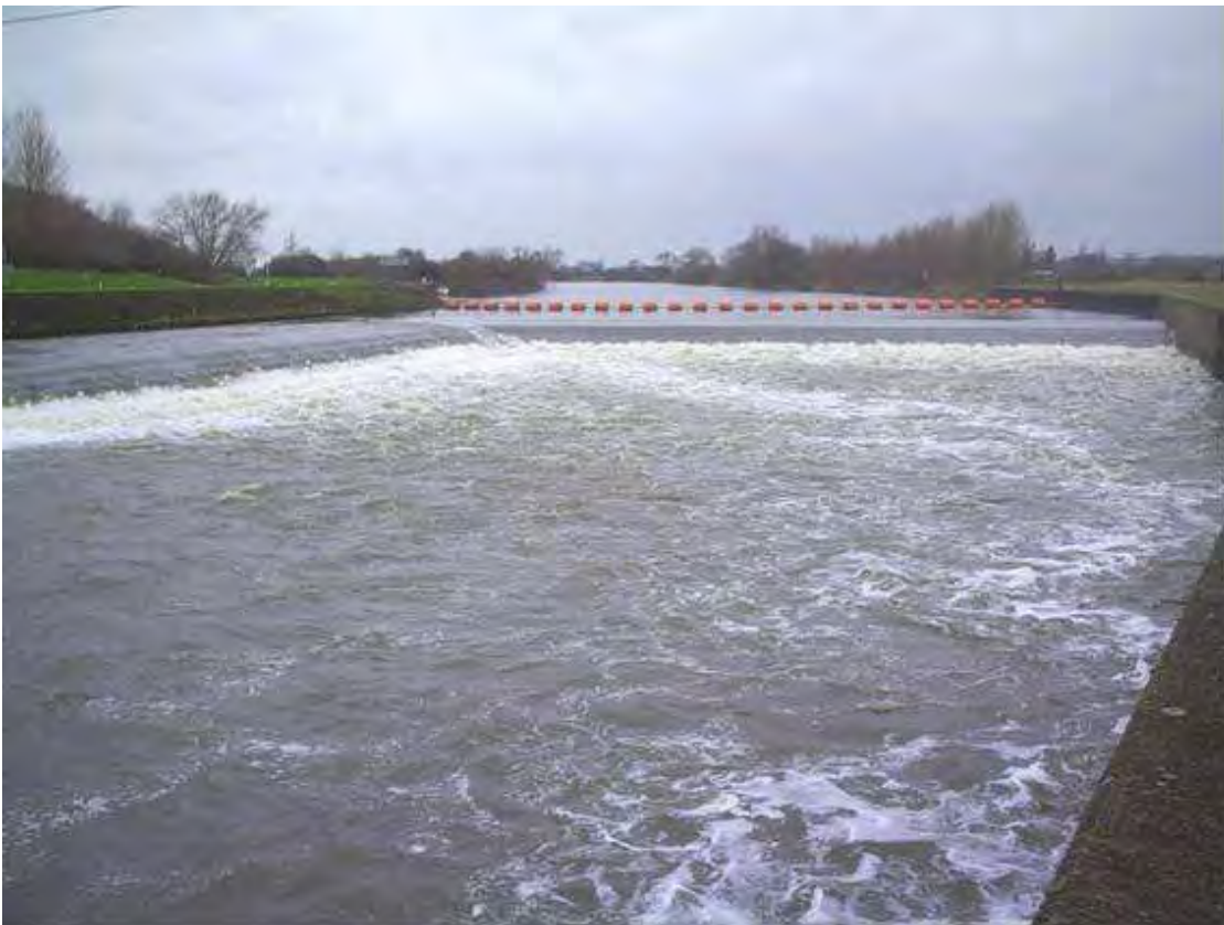
Plate 30 Hazelford Weir on the River Trent (source: HIFI)
