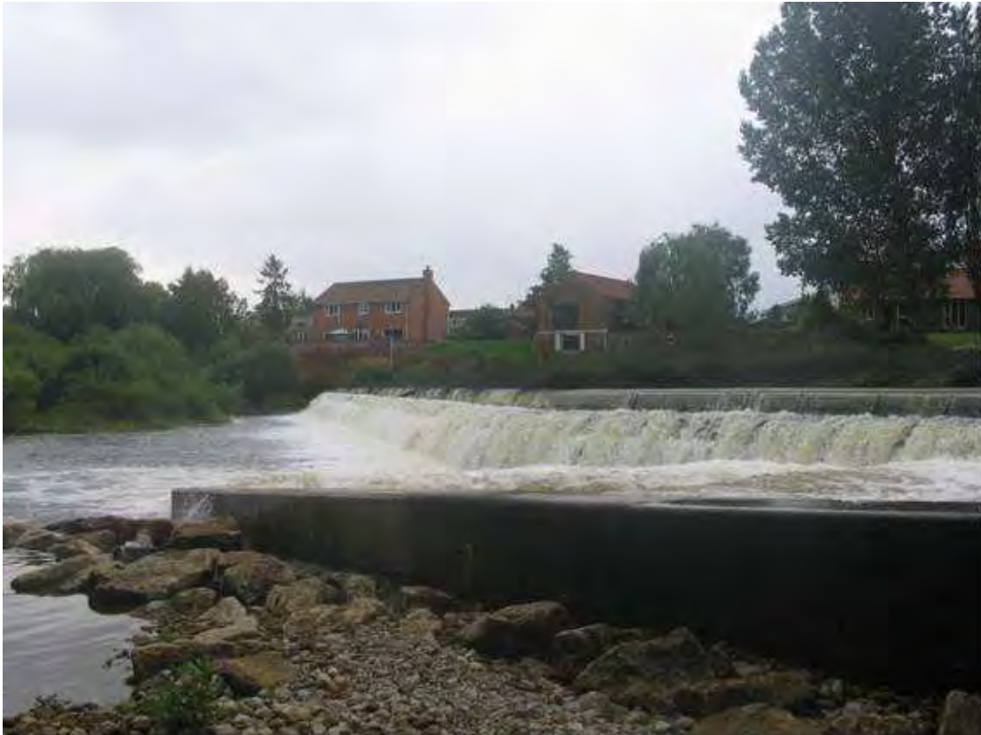
Plate 12 Boroughbridge Weir on the River Ure (source: HIFI)
