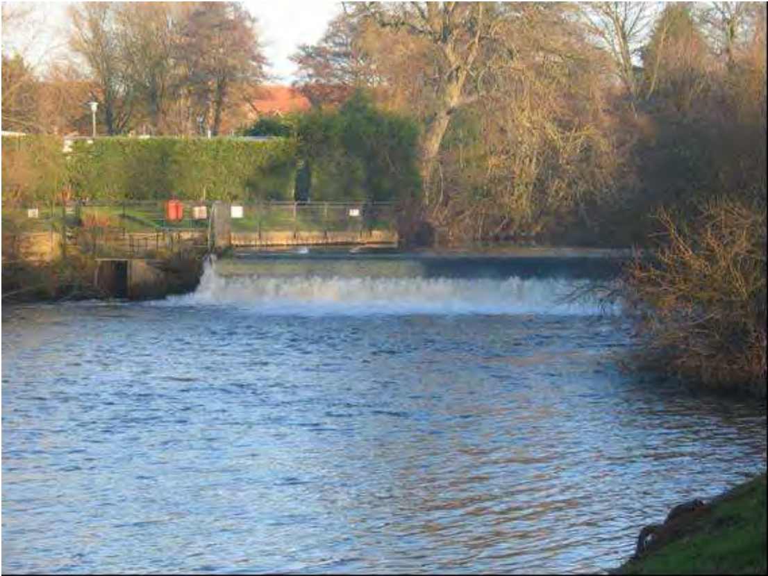
Plate 8 Stamford Bridge Weir on the Yorkshire Derwent (source: HIFI)
